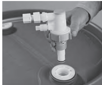
2. Insert coupler into drum insert assembly.
